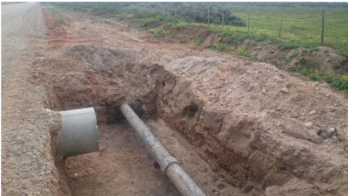
Main waterline to Lambertsbay affecting protection works of pipe culvert
