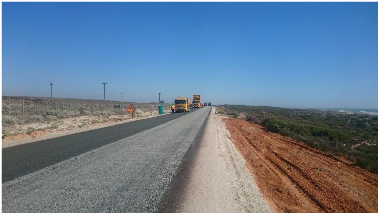
Putting the permanent pavement layers down on Main Road 538 near Muisbosskerm, Lambertsbay
